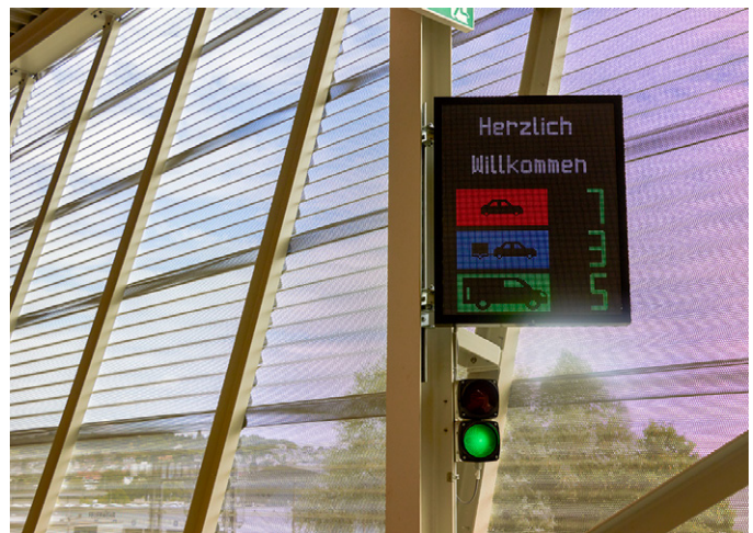
A guidance system provides information about the occupancy of spaces according to three vehicle categories.
