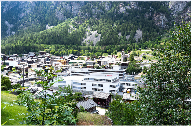
The Scintilla AG plant is located in St. Niklaus in the Mattertal valley at 1120 metres above sea level.
