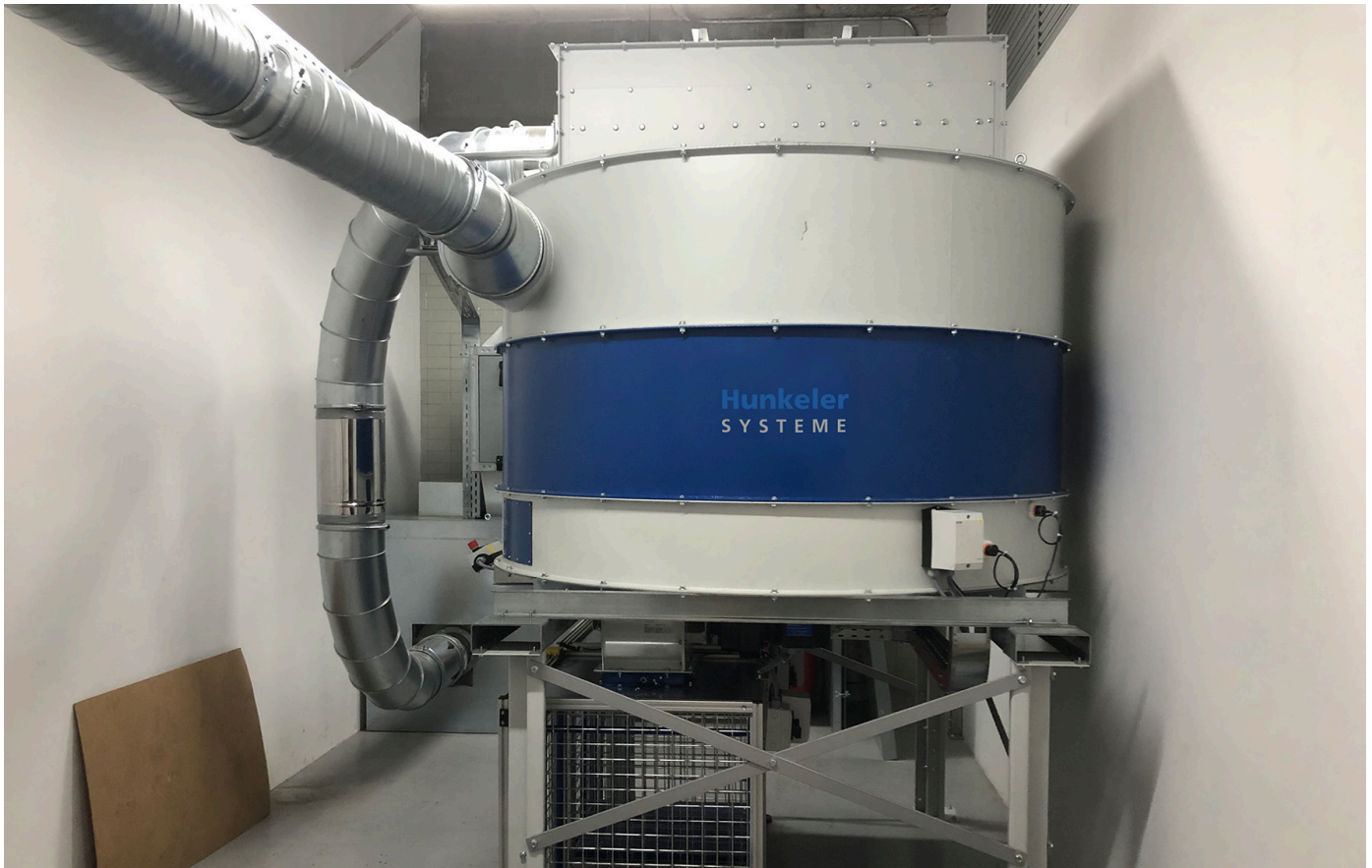
A fine filter guarantees the required air quality of a maximum of 0.1 milligrams residual dust content per cubic metre.
