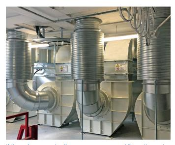
If there is no production on one or several lines, the automatic switch-off puts the corresponding fans in stand-by mode.
