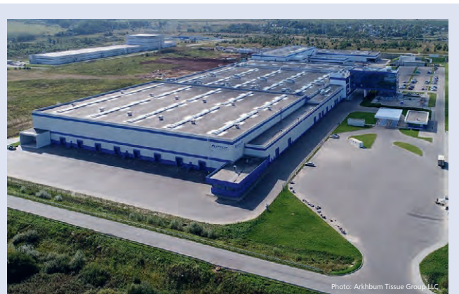
The Arkhbum Tissue Group LLC put their new production facility at Vorsino Industrial Park into operation in September 2020..
