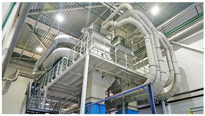
As the extraction and compaction plant is installed on two levels, optimal use of the available vertical space is made.
