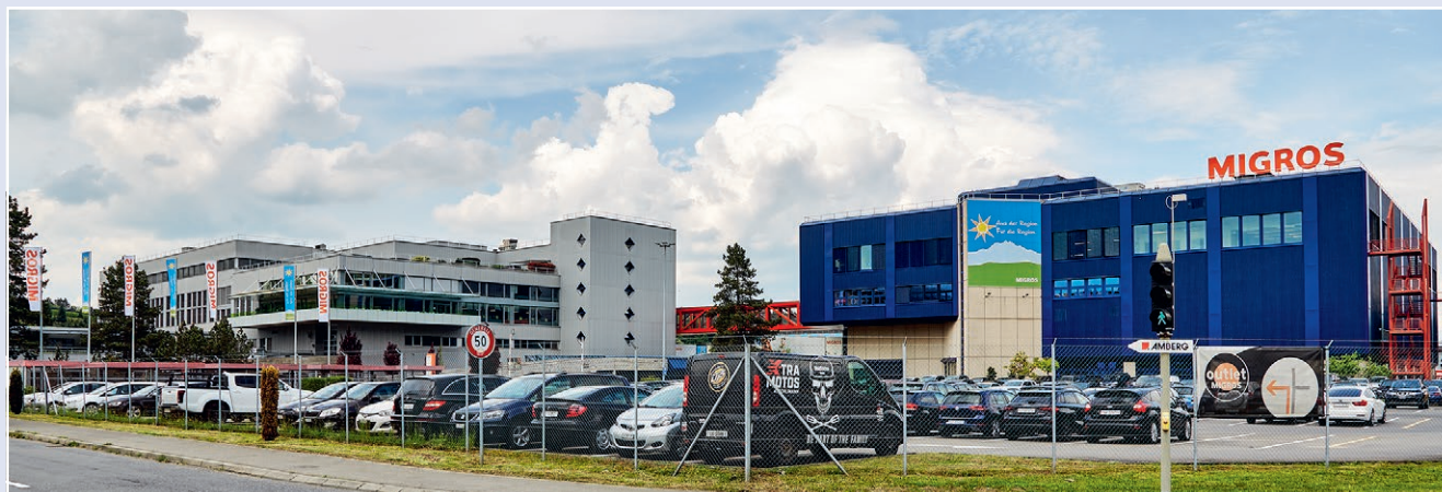
The supermarket branches and restaurants of the retailer throughout central Switzerland are supplied with products every day from the distribution centre in Dierikon.
