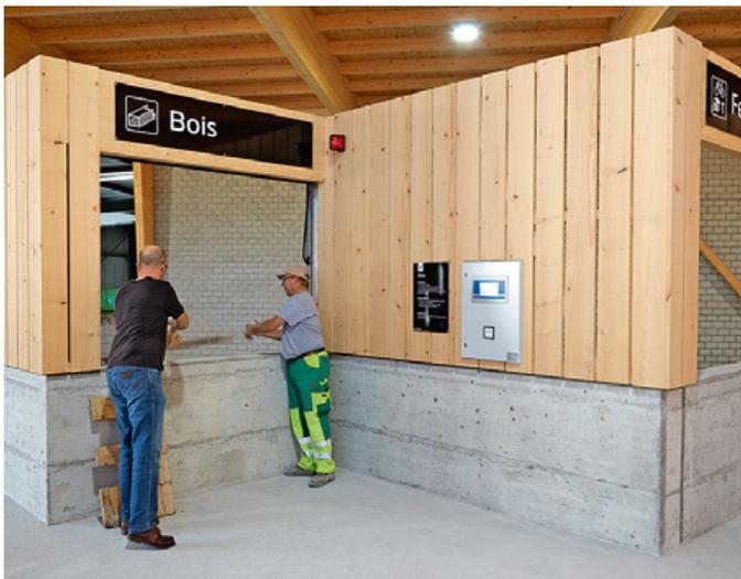
Wood and mineral waste/unburnable waste is disposed of through large sized gates in the container. The containers stand on scales, the badge is debited according to the material and the weight.
